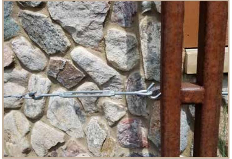
**A cable and welded steel trellis for espaliered trees**
