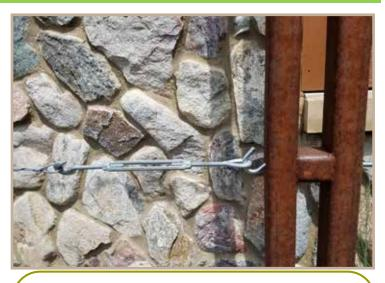
A cable and welded steel trellis for espaliered trees
